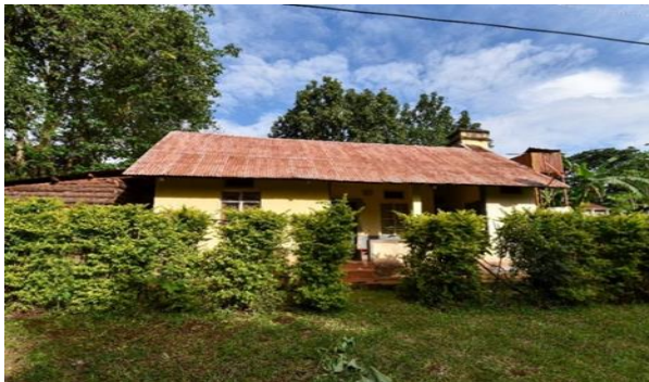
Staff housing to be renovated
